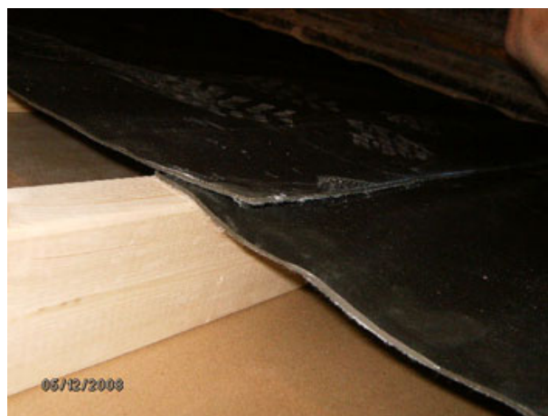
Figure 2. Example of Installation of dB-3™ - detail.
