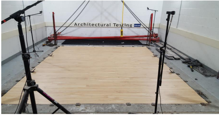
Source Room View of Test Specimen Installation
