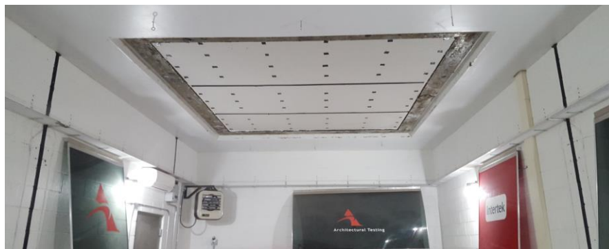
Receive Room View of Test Specimen Installation
